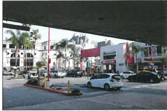
2C. EXISTING STRUCTURE, LOOKING EAST
